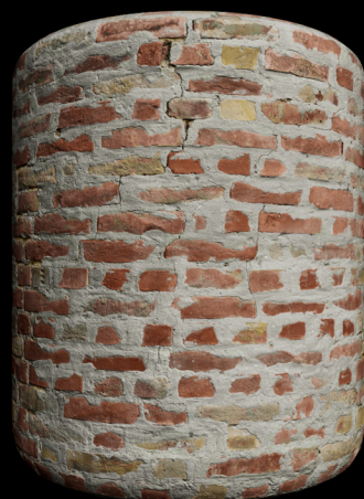
Bricks & Sloppy Mortar 03
